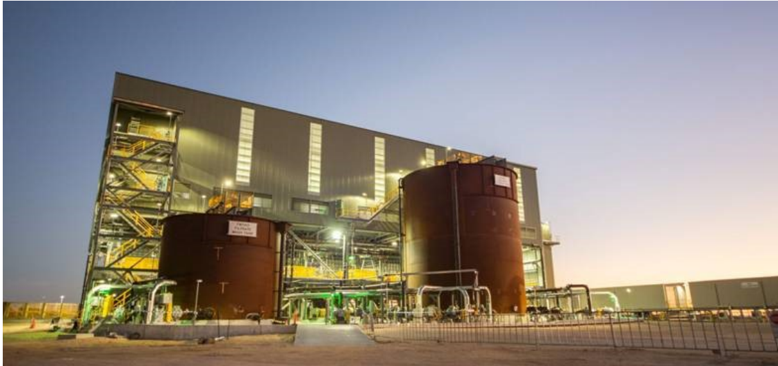
Figure 8. Refinery – Outside Building.
